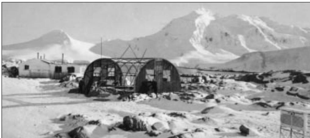
1944 - with Bransfield House nearing completion, the next task was to erect the ex-Army Nissen hut. Photo: Gwion Davies. © British Antarctic Survey.
